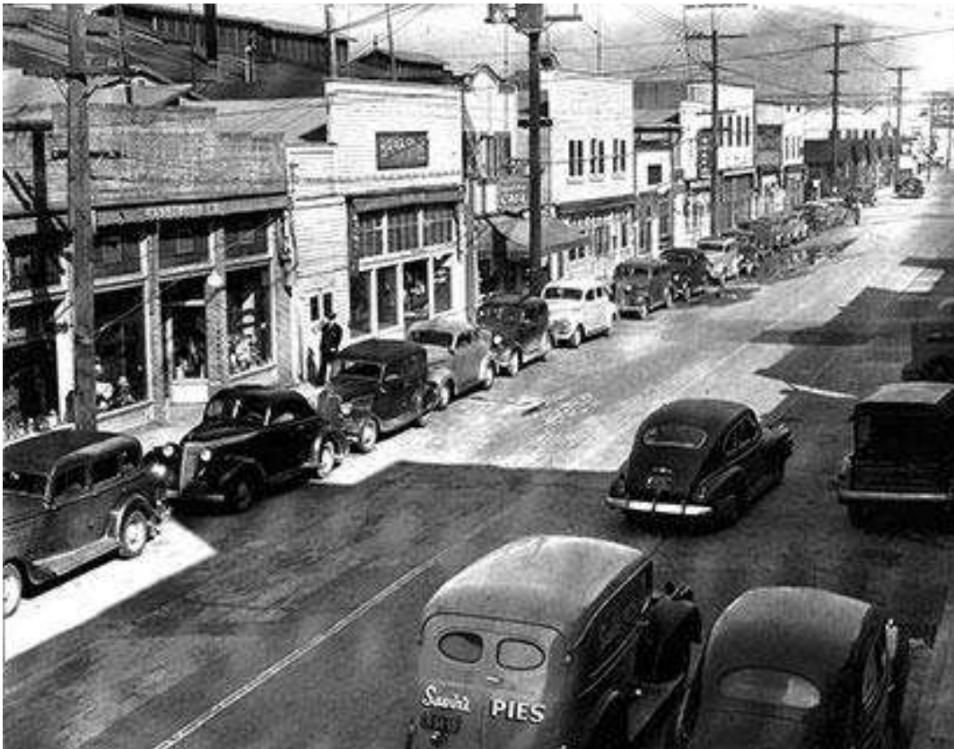
Tuna Street - the Main Commercial Street on Terminal Island
